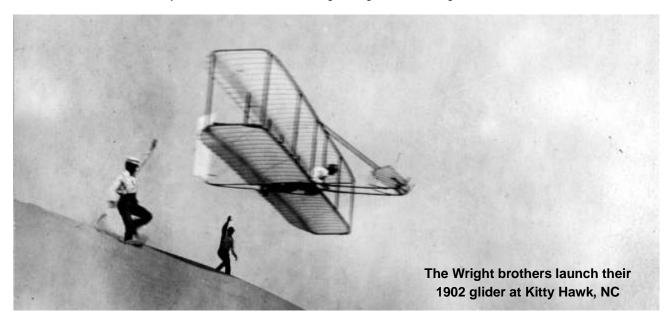
The aircraft was unstable in pitch. The computed a time to double amplitude was about 1.8 seconds. This means if you have a pitch up of five degrees and do not correct it, in 1.8 seconds it will be at ten degrees. If you still do nothing to correct it the pitch up will reach twenty degrees, and so forth.
