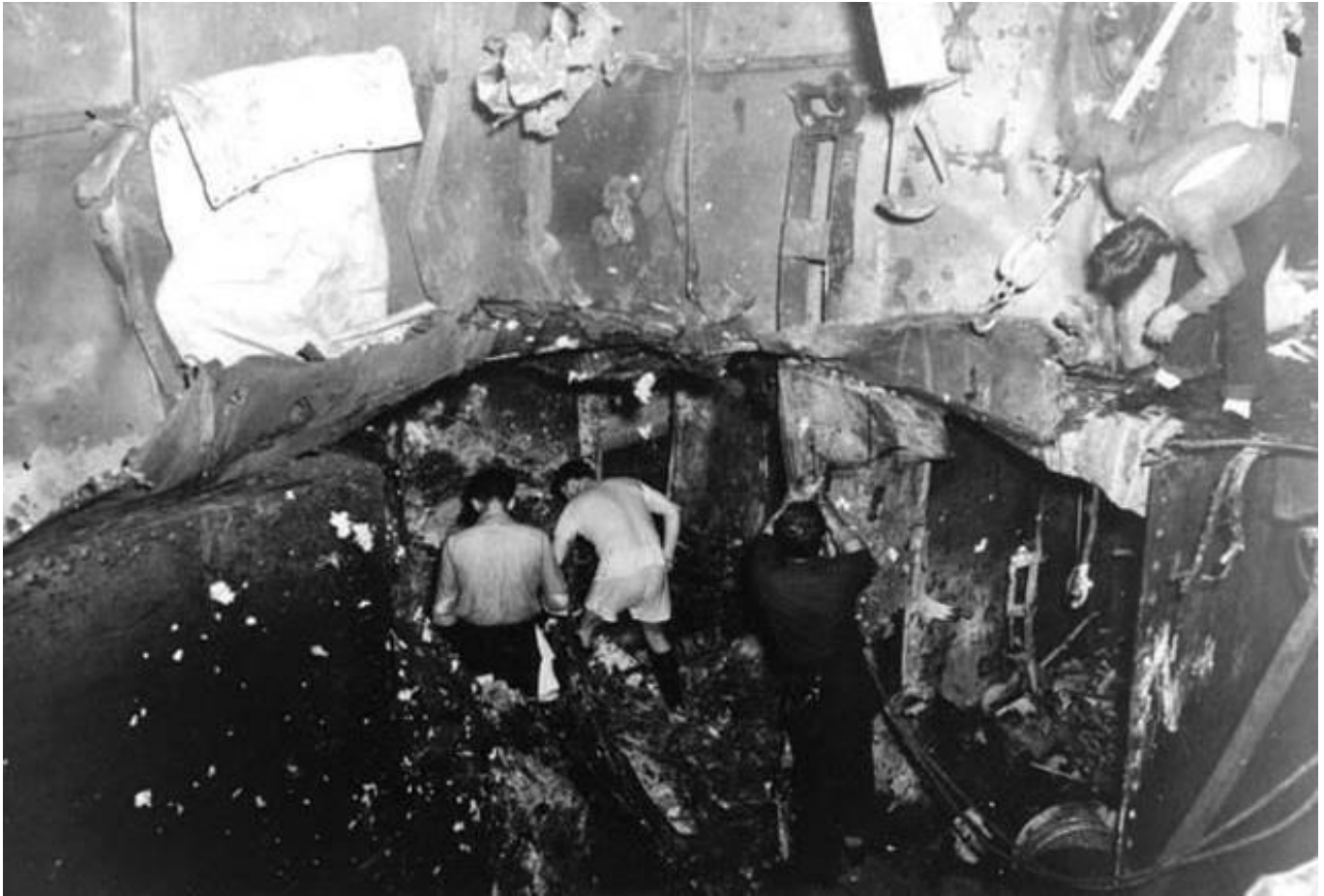
Bomb damage on Yorktown's third and fourth decks, copied from the war damage report, 1942.
