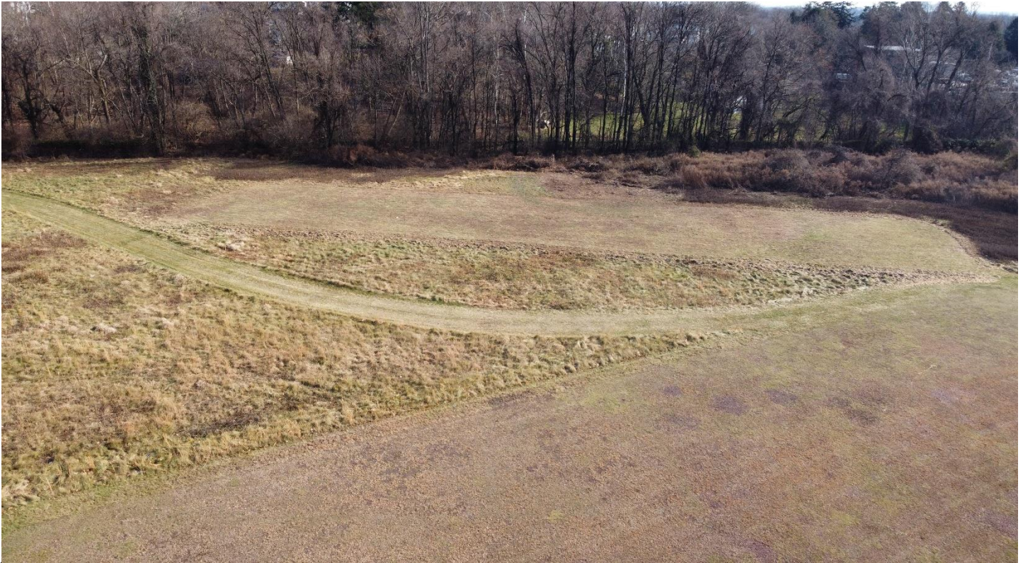
The new South Runway takes shape at Elwyn Field
