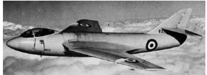
*Hawker 1081 Hunter forebear with aft fuselage exhaust and wing fences. Wing aerodynamics was a real challenge approaching Mach 1.*
